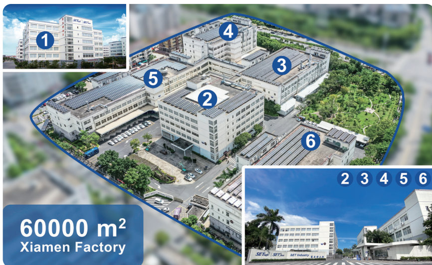
SETsafe | SETfuse Industrial Park
